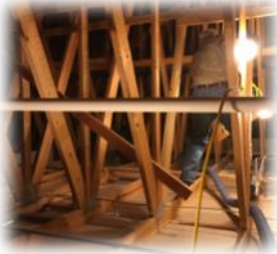
Insulation blown into the Attic
